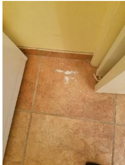
Flooring/Baseboard Taken on: 2017-03-11 16:49:52 Taken at: 40.62384946, -111.87139269 Image
