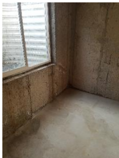
Wall/Ceiling Taken on: 2017-03-11 16:53:28 Taken at: 40.62387083, -111.87150382 Image
