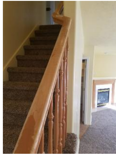
Railing/Banister Taken on: 2017-03-11 16:23:07 Taken at: 40.62395069, -111.87151184 Image
