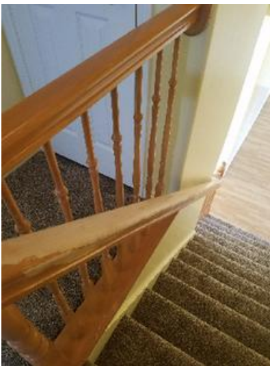
Railing/Banister Taken on: 2017-03-11 16:23:41 Taken at: 40.62393293, -111.87148837 Image
