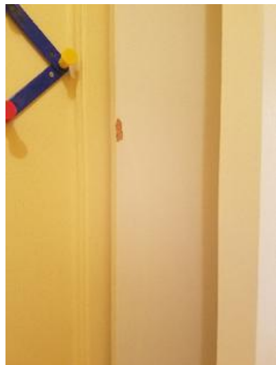
Wall/Ceiling Taken on: 2017-03-11 16:50:58 Taken at: 40.62387972, -111.87145206 Image
