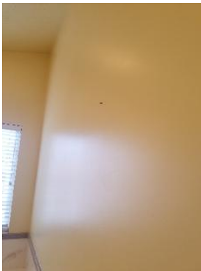
Wall/Ceiling Taken on: 2017-03-11 16:38:49 Taken at: 40.62398679, -111.87147587 Image
