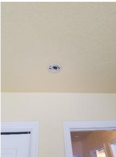
Smoke/CO Detector Taken on: 2017-03-11 16:27:09 Taken at: 40.62390802, -111.87151126 Image
