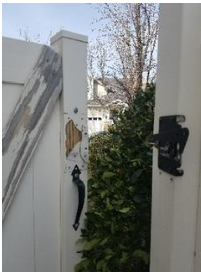
Fence/Gate Taken on: 2017-03-11 16:11:21 Taken at: 40.624137, -111.8710648 Image
