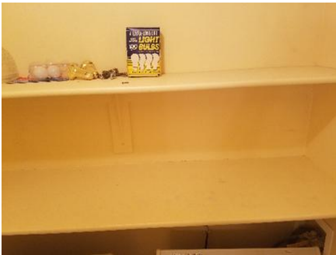
Wall/Ceiling Taken on: 2017-03-11 16:50:06 Taken at: 40.62386265, -111.8714145 Image
