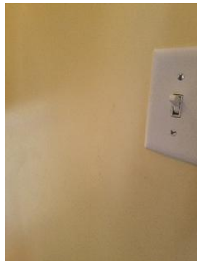
Wall/Ceiling Taken on: 2017-03-11 16:23:58 Taken at: 40.6240613, -111.8710648 Image
