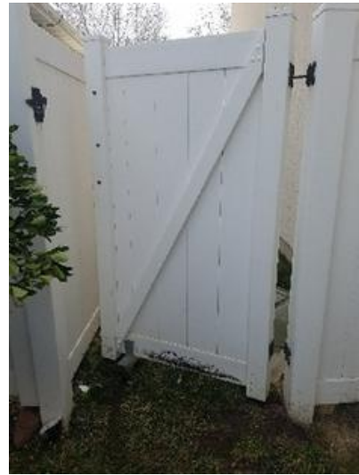
Fence/Gate Taken on: 2017-03-11 16:11:12 Taken at: 40.624137, -111.8710648 Image
